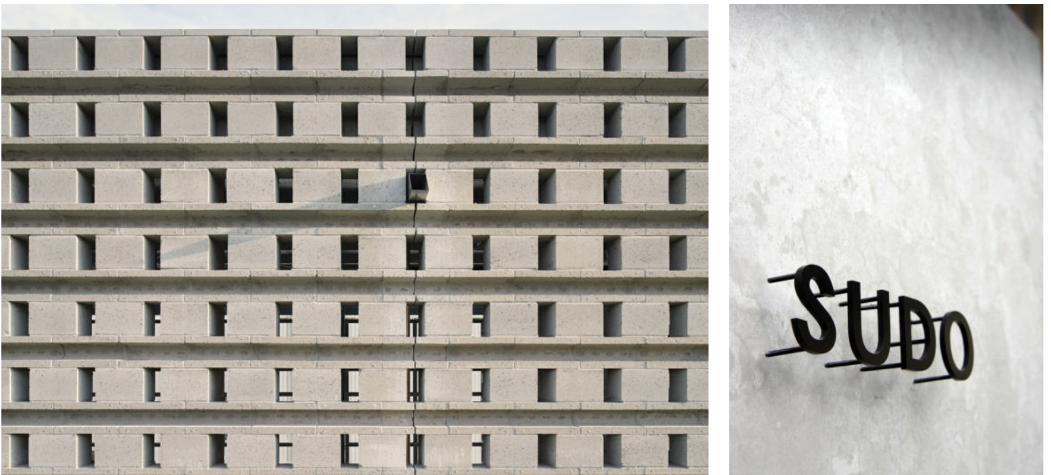
EW-04 - EXTERNAL PATTERN MASONRY BLOCK WALL SIG-01 - METAL PIN HUNG SIGNAGE WITH LIGHTING
